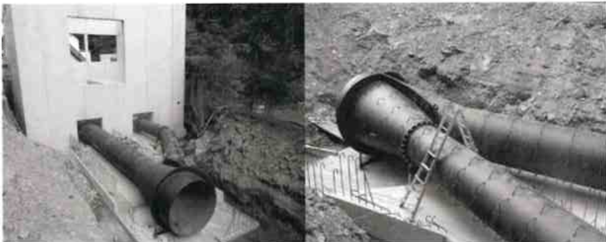
Since 2012, GUGLER Water Turbines GmbH (Austria) uses the system ZINGA 1 x 60 µm DFT + Zingatarfree 2 x 100 µm DFT as a basis to protect the underground parts of water tubes. This system will provide a protection that accords to the ISO 12944-6 test results predicting a life expectancy of >15 years on structures immersed in soil.
